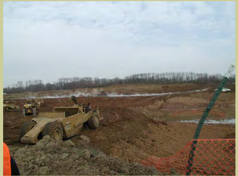
Lambert Airport Construction
