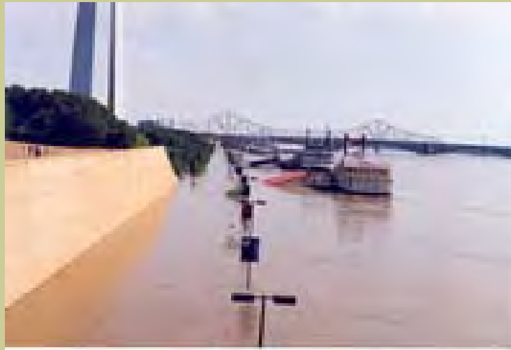
Downtown Flood Wall near St. Louis Arch
