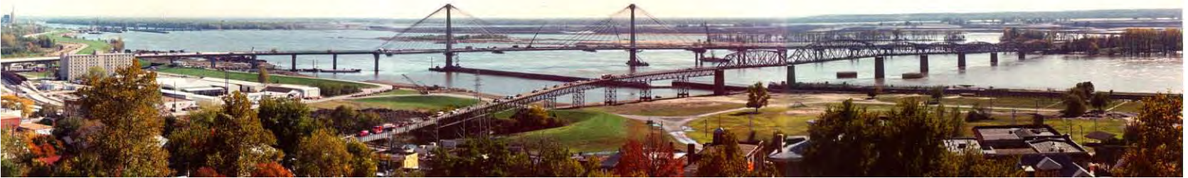
Panoramic View of Clark Bridge near Alton, IL
