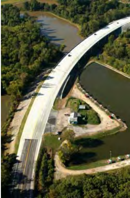
Highway 21 at Butler Lake
