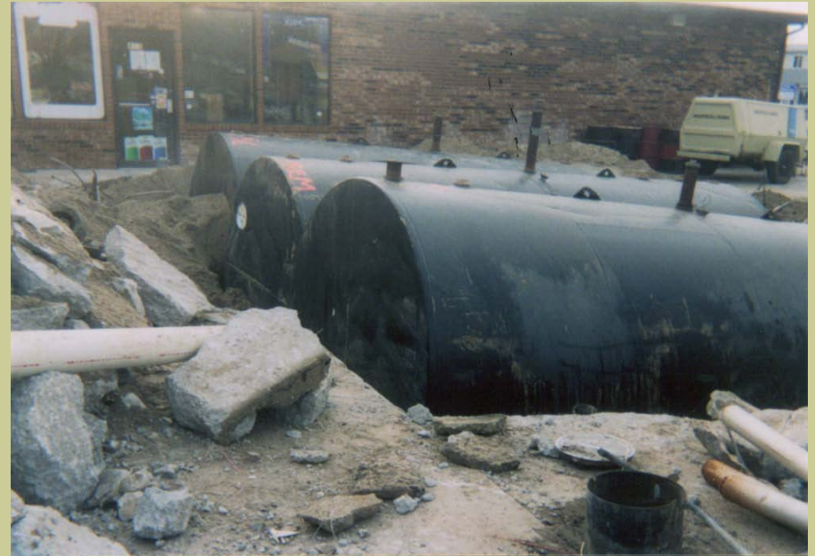
Underground Storage Tank Clean-Up and Removal
