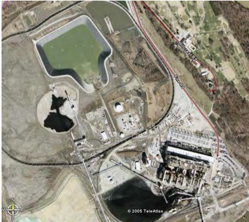
Lower Meramec River Wastewater Treatment Plant
