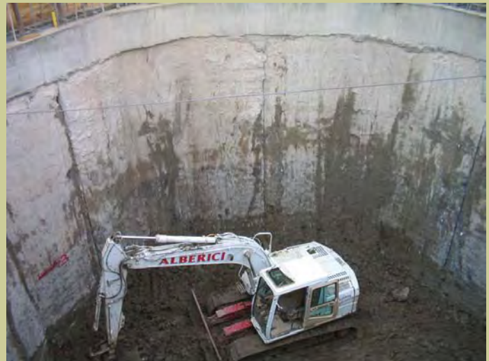
Lower Meramec Treatment Plant Construction
