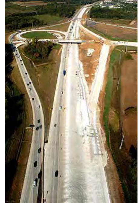
Hwy. 40 & K Interchange
